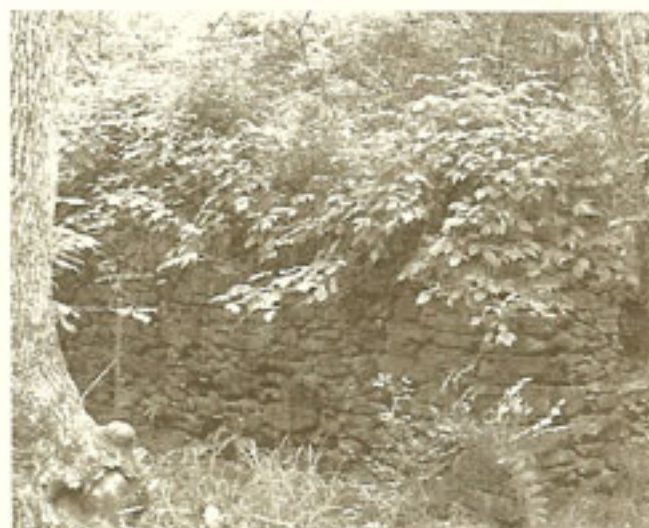
Remnants of the mill's stone foundation.
